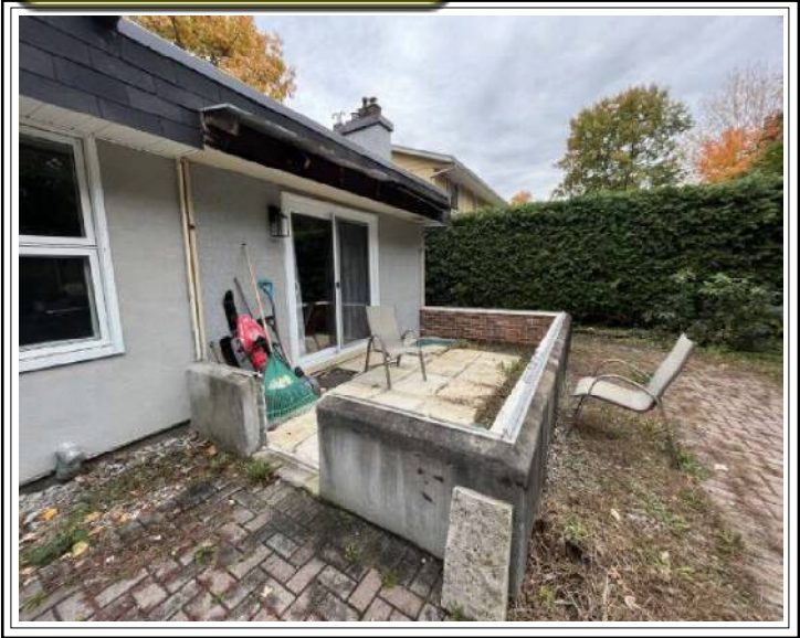
originally glass solarium / glass has been removed
